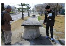
**Fig. 2** Raised manholes caused by soil liquefaction (Urayasu City).
